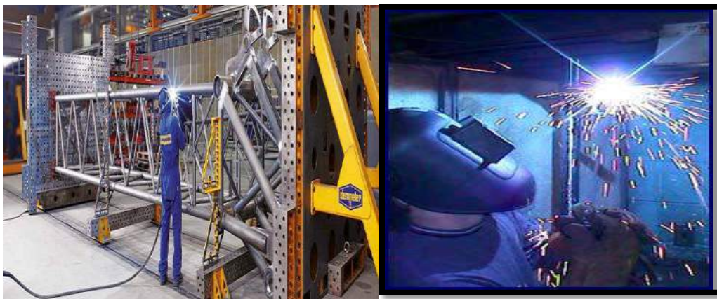
Welding above shoulder height
