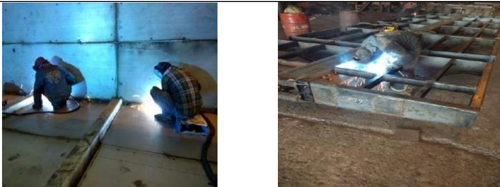
Welding at ground level
