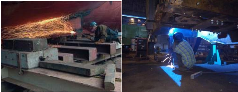
Welding in constrained spaces
